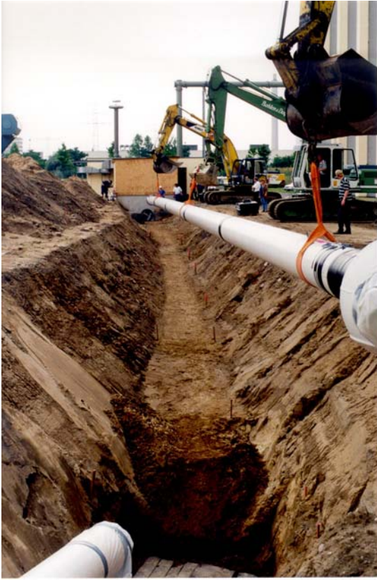
Fig. 2: Directly buried version of GIL
