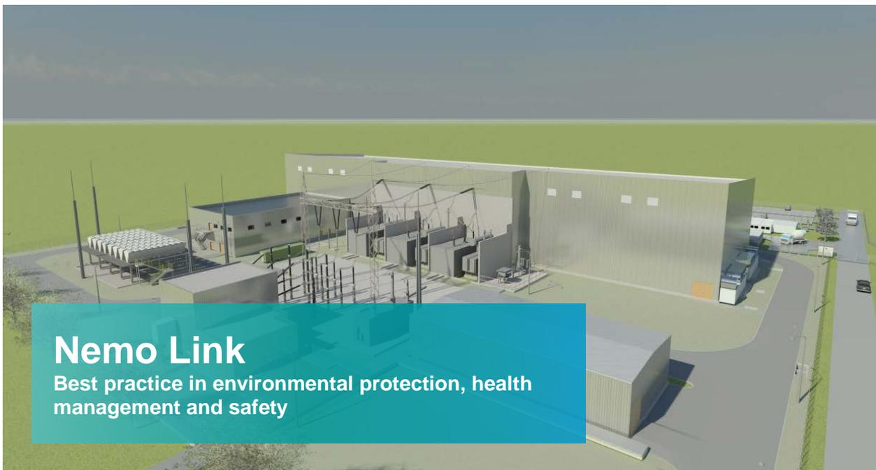
In November 2017, the HVDC project “Nemo Link” connecting United Kingdom with Belgium received the Sword of Honour award 2017 ([Press Release](#)) for the UK part. It is the first DC link in modular-multilevel voltage-sourced converter technology (HVDC PLUS) at  $\pm 400$  kV DC configured as symmetrical monopole for a power transmission capacity of 1,000 MW. Siemens received the contract for the converter stations from Nemo Link Ltd.
