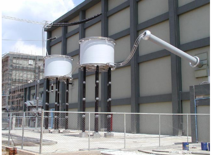
Fig. 7: Example for Series Connection of Dry-Type Smoothing Reactor Coils
